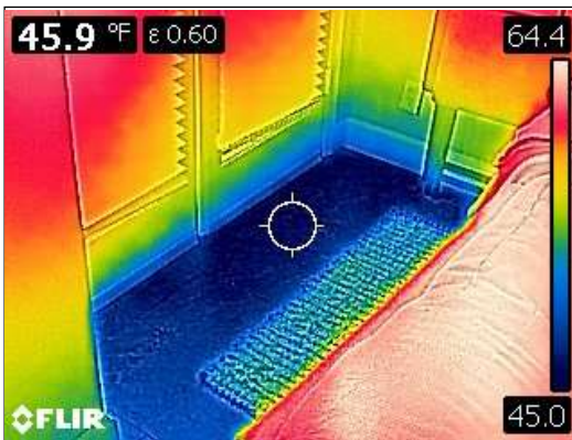
Bedroom floor infrared scan
