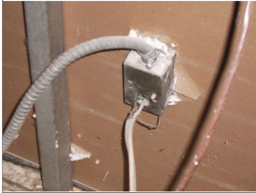
Wires pulling out the dining wall receptacle
