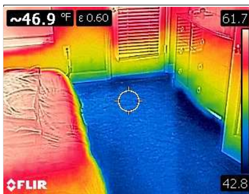
Bedroom floor infrared scan
