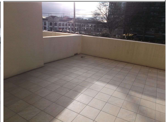
Drainage hole in condo balcony wall
