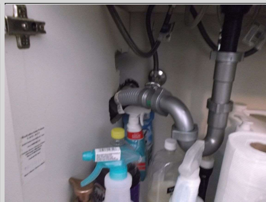
DIY drain pipe repair
